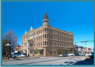
Chiquola Hotel Anderson, SC (Agnew Rincon Architects)
